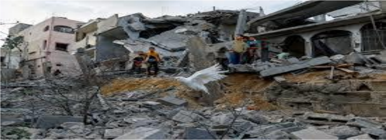
Figure 3: Debris of houses destroyed in Israeli strikes, in Khan Younis in the southern Gaza Strip October 11, 2023.
